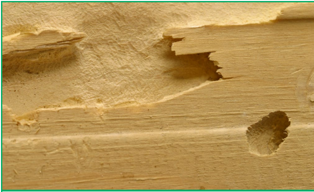
Figure 4. Old house borer damage. Photo by Michael Merchant.
