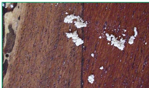
Figure 1. Frass from wood boring beetles. Photo by Wizzie Brown.
