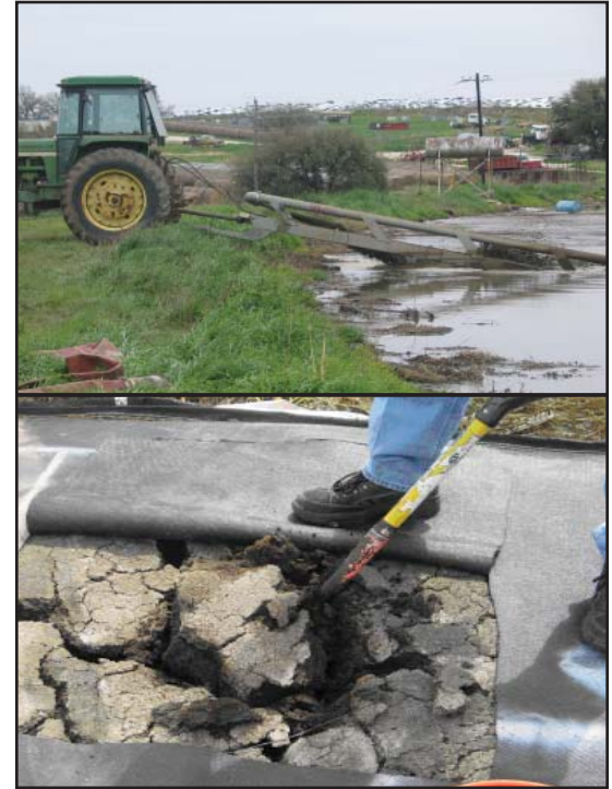
Fig. 3 (top): Chopper pump mixing the lagoon Fig. 4 (bottom): Residual solids in dewatered Geotube®
