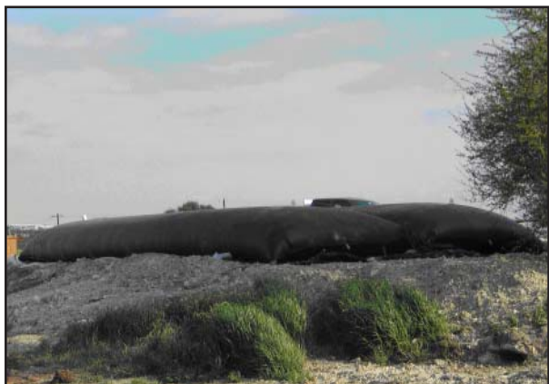
Fig. 2: Filled Geotubes®
