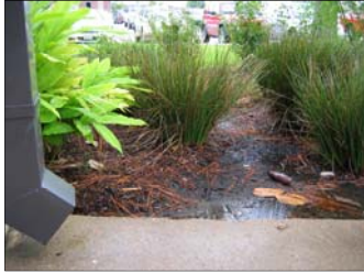
...from a roof
