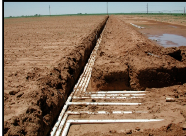
Figure 2. Installing water lines to different SDI zones, TAES, Helms,
